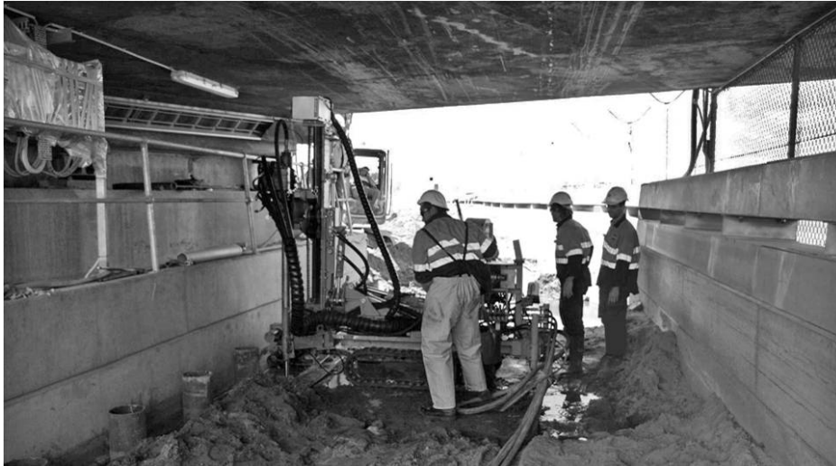
Figure 5: Implementation of a special mini rig for low head areas
