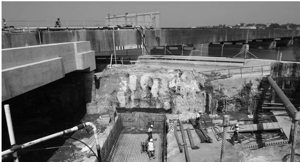
Figure 6: Excavation and construction of SWSOOS support structure after jet grouting
