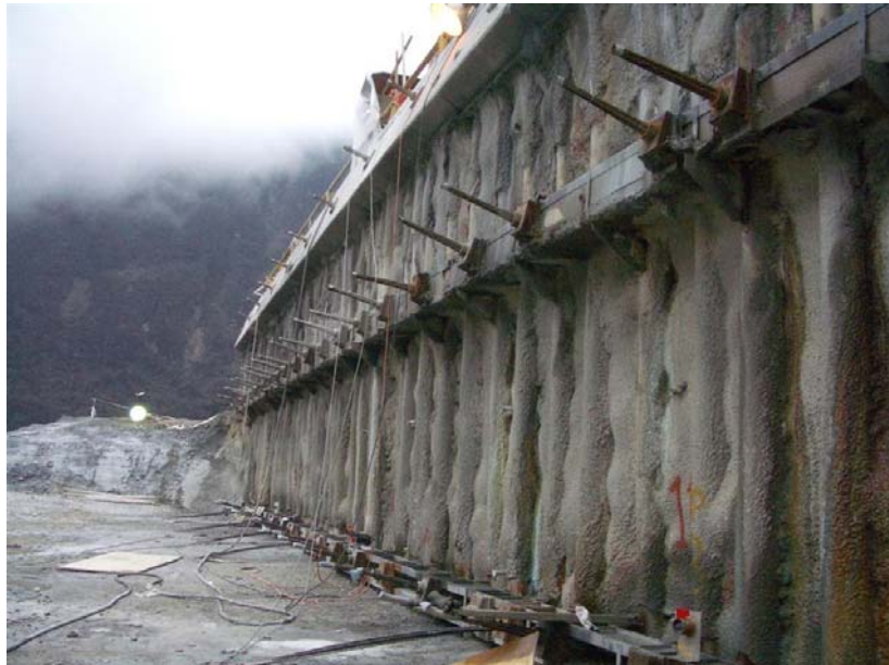
Photo 2 – Piled wall after anchor installation third row
