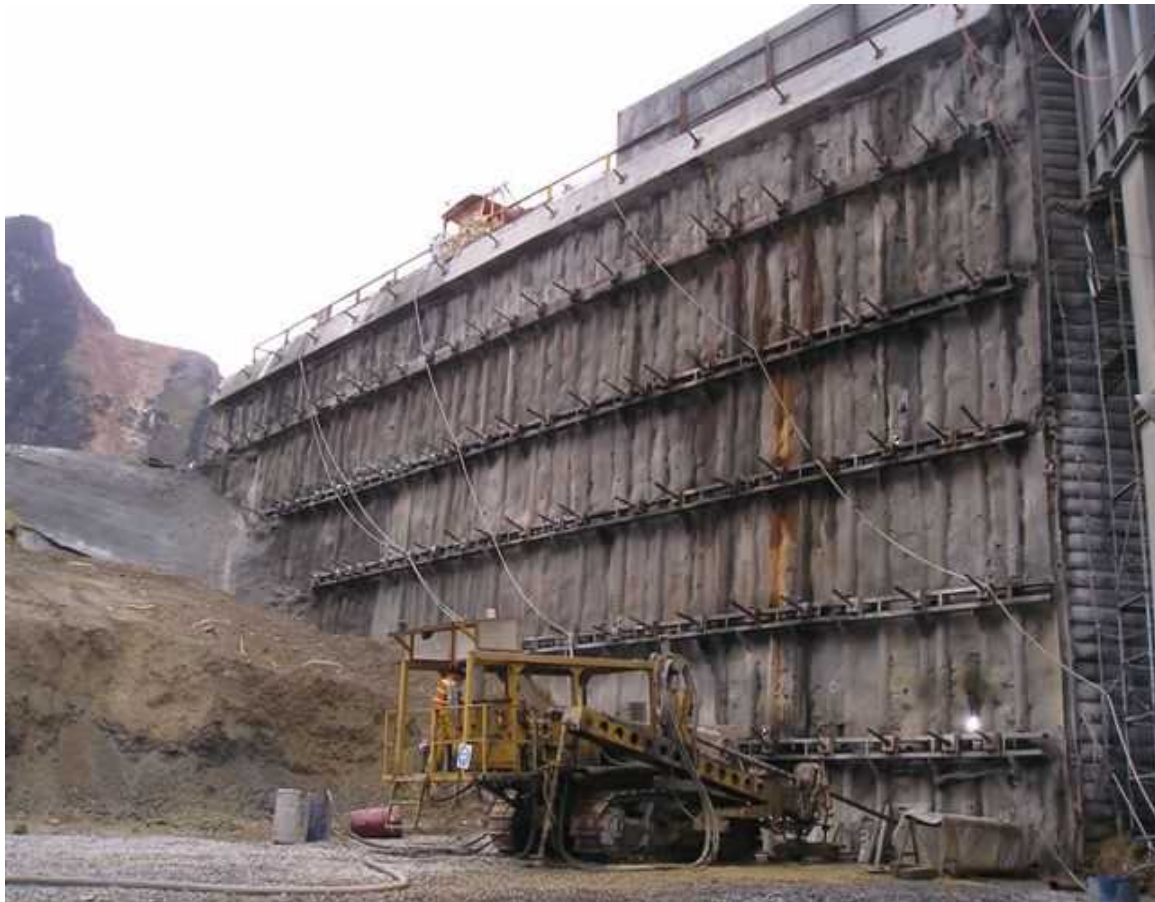
Photo 4 - Freeport Mine anchored piled wall to Crusher 7 Dump Slab
