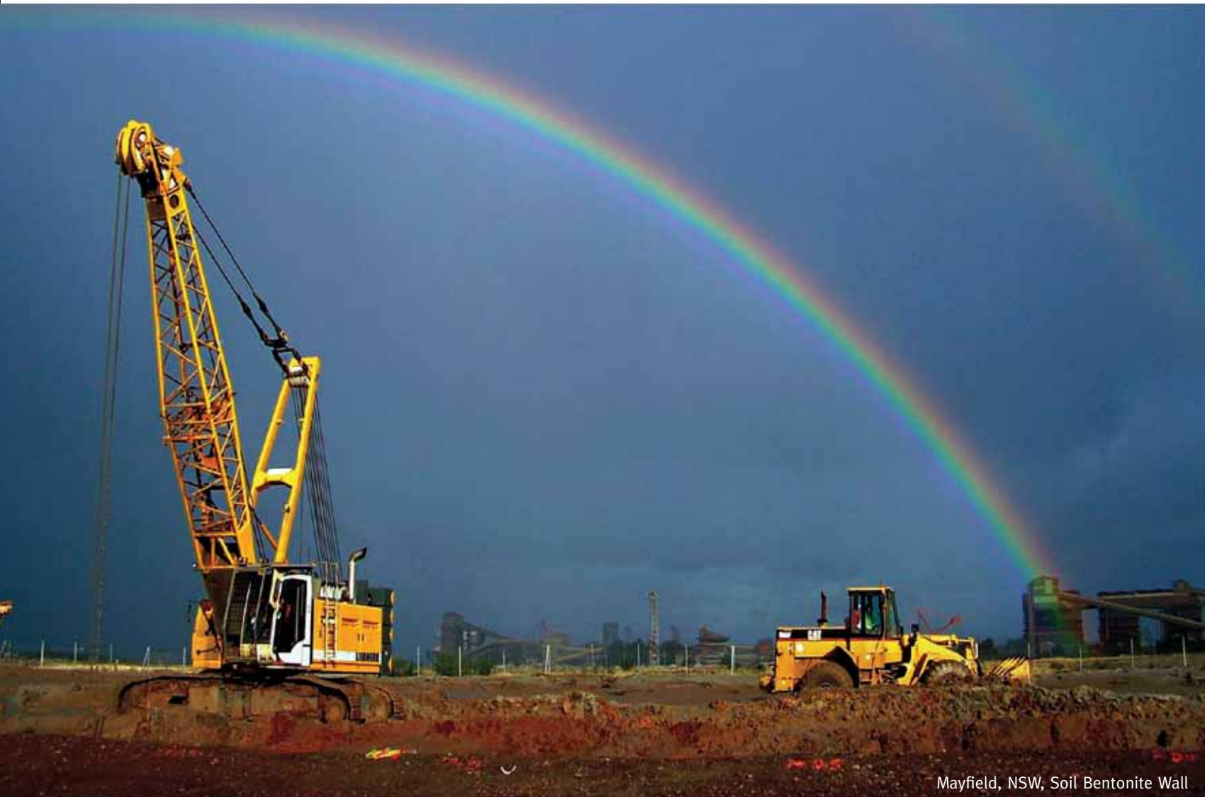
Mayfield, NSW, Soil Bentonite Wall
