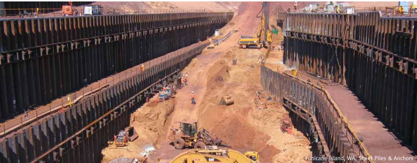
Funicane Island, WA, Sheet Piles & Anchors
